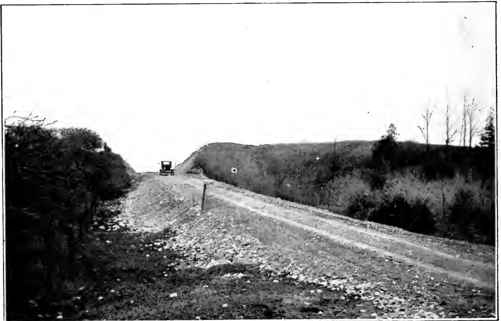
HURON COUNTY ROAD Grade reduction in Grey Township.
